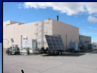
DG Test Location
