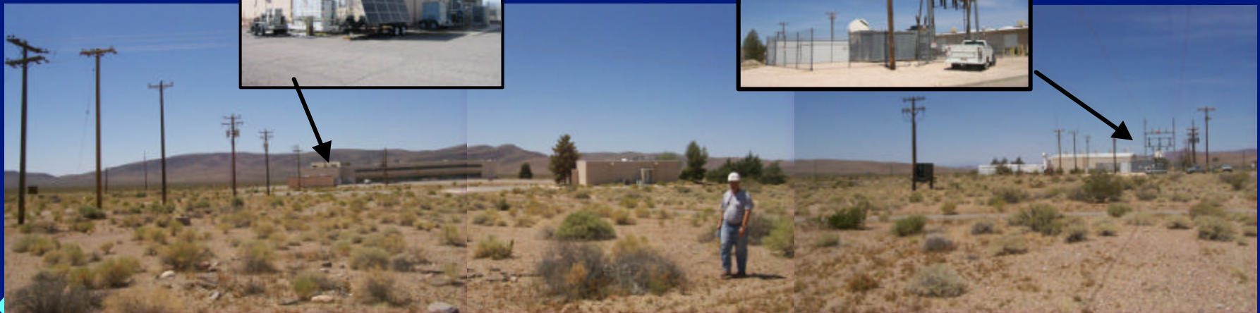
Feeder 25-1202 at Area 25 of Nevada Test Site
