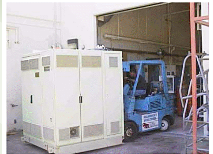
25kW SOFC system being installed at NFCRC
